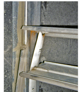
TAMCO Series 1000 SW assembled out of square
