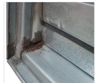
Accumulation of blade fragments
