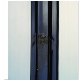
Series 1000 SW assembled out of square
